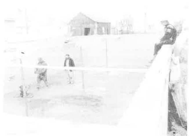
Working on the basement for St. Mary's Church, 1970-71.
