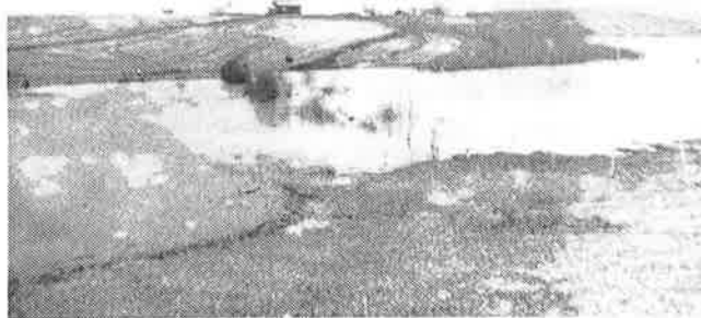
1955: Kildrum road flooded
