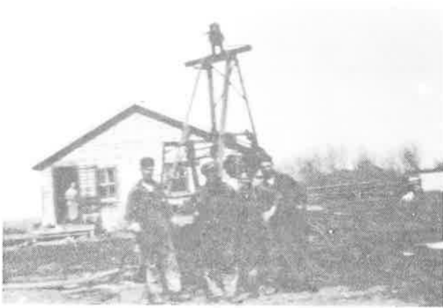
Charles Stahl and the well drilling machine.
