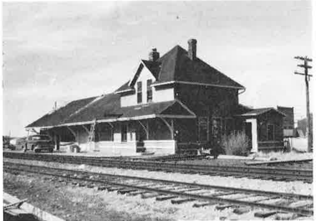
Bruno Station -- demolition has already begun
