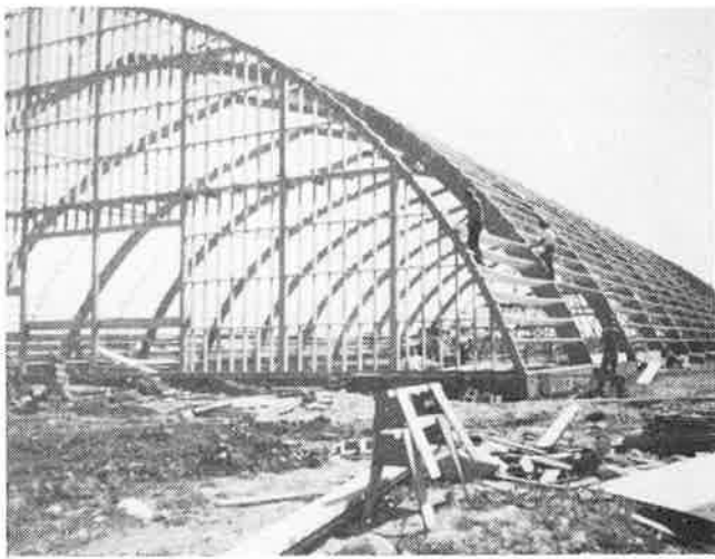
New skating rink under construction
