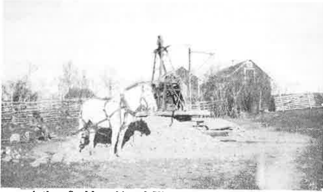
Arthur Serblowski and Slim with well digging outfit
