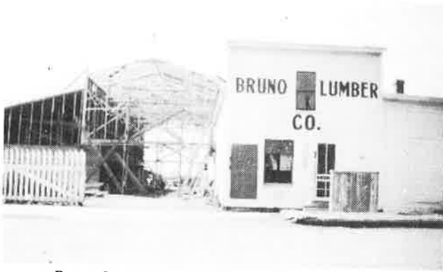
Bruno Lumber Co. addition under construction
