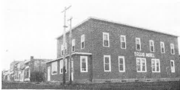
Bruno Hotel after renovation
