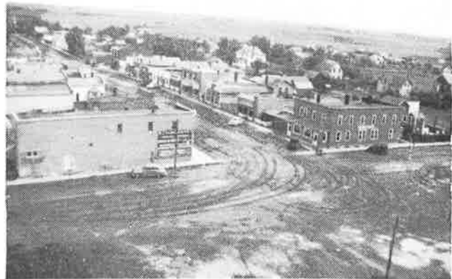
Bruno - taken from the top window of the Searle Elevator, while it was being built, 1950.
