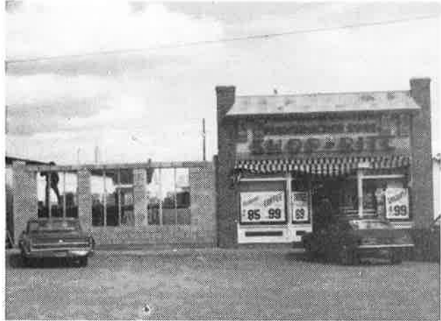
Renovations to Pulvermacher Bros. Shop-Rite
